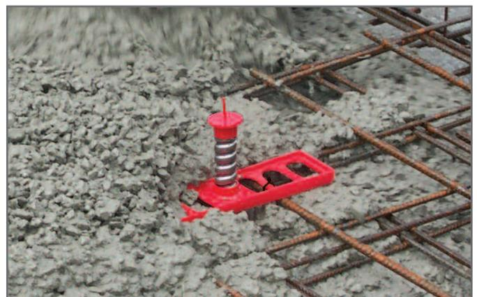
The installation-kit is attached firmly to the reinforcement and remains in vertical position. After smoothing the concrete surface it is very easy to discover the anchoring point by the flexible pin of the marking plug.
